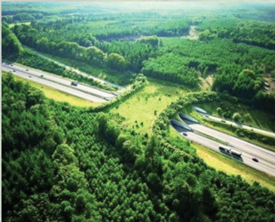
A Wildlife Crossing at Highway A50 in the Netherlands
